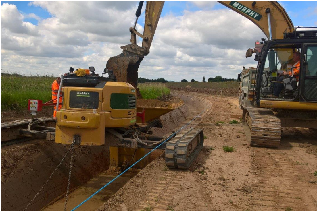
Plate 5-10 Example of Open Trench Technique, Sofia offshore wind farm (2022)
